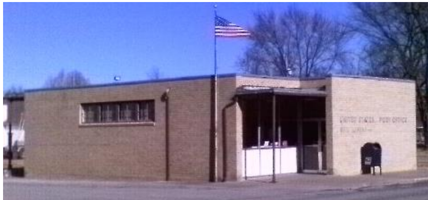
Weir Post Office
