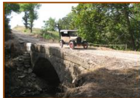
Figure 4 Timber Creek Bridge
