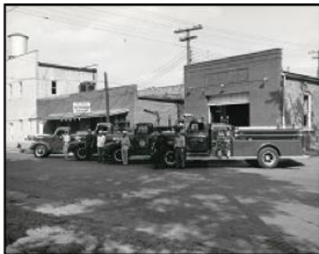
Figure 4 Neodesha, Kansas Fire Station & Equipment
