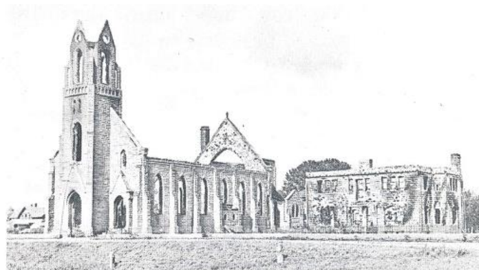
Figure 14 The Liebenthal Church after the fire.
