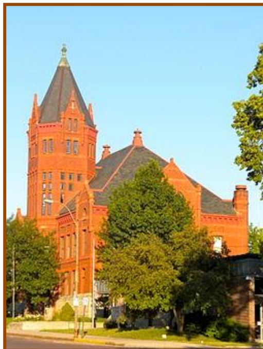
Figure 7 Marshall County Courthouse
