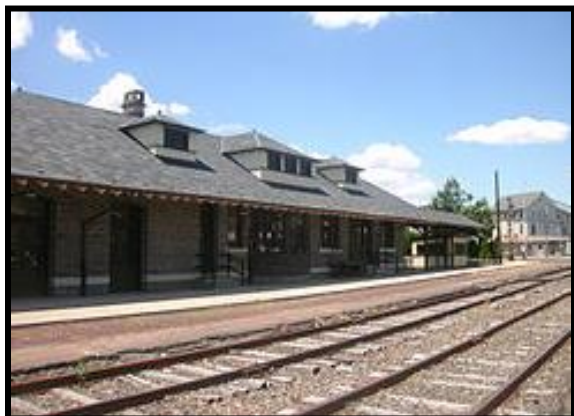
Figure 5 Quakertown Passenger and Freight Station
