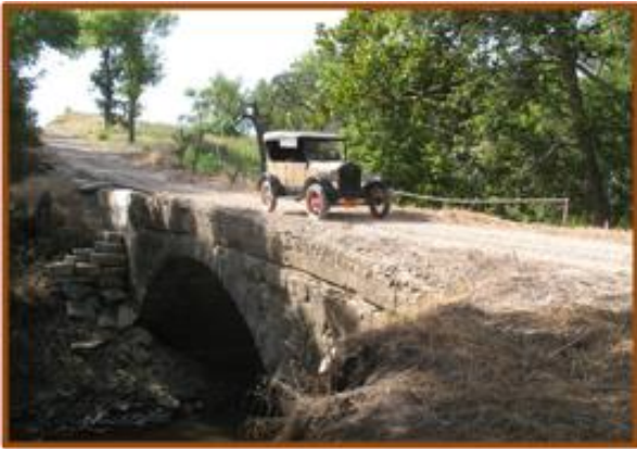
Figure 6—Timber Creek Bridge built in 1908
