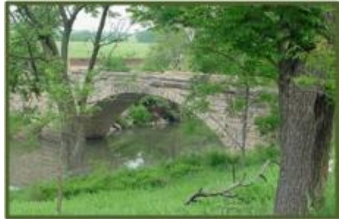
Figure 7—Fox Bridge built in 1910
