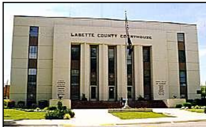
Figure 5 County Courthouse in Oswego
