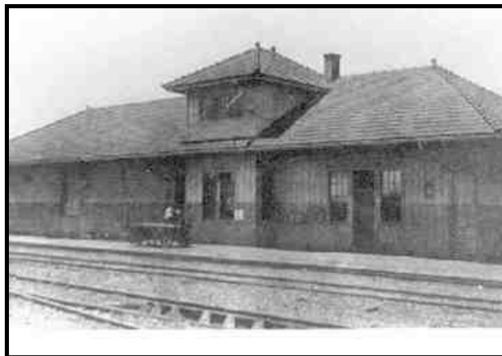
Figure 3--Railroad Depot Moran Kansas
