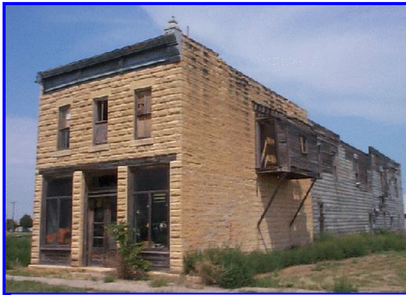
Figure 3--Stone Structure built in 1880
