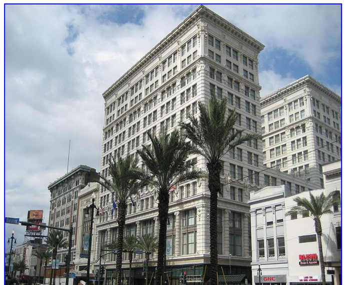
Figure 2--Maison Blanche Building Canal Street
